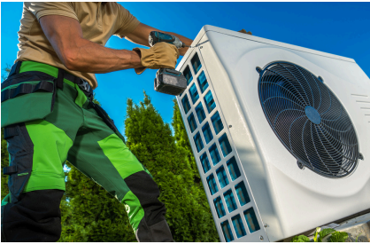
HEAT PUMP INSTALLERS
